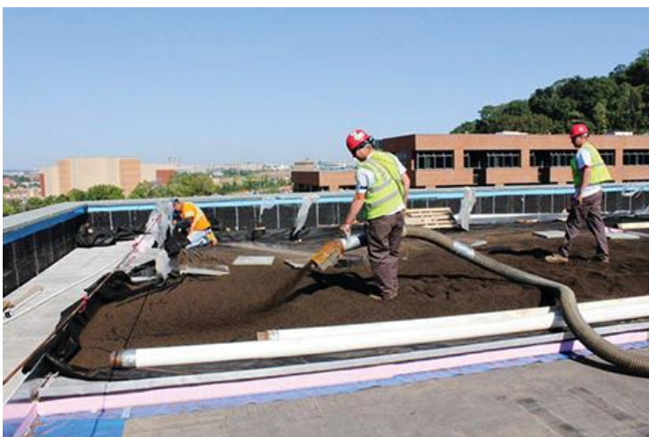
An example of an application for XPS include within vegetated roofing assemblies. Photo courtesy Owens Corning
