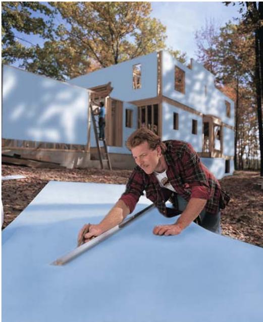
*Figure 1: Installation of sheathing insulation*
