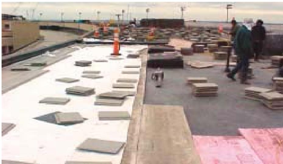
**Figure 4.** Dallas/Fort Worth reroofing project with Owens Corning Foamular XPS insulation.
