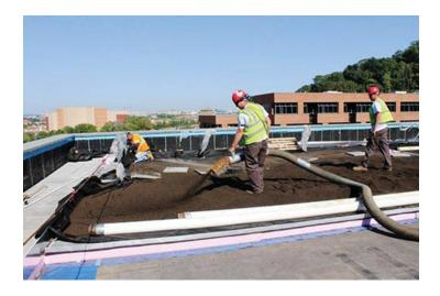
An example of an application for XPS include within vegetated roofing assemblies. Photo courtesy Owens Coming
