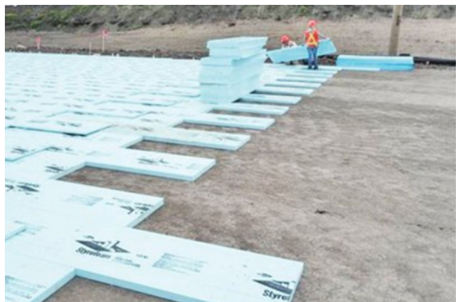
Highway geofoam application. (Courtesy of DuPont.)
