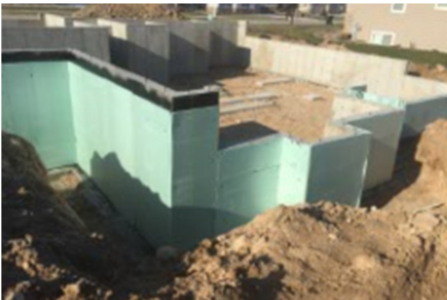
Below-grade wall application. (Courtesy of Kingspan.)
