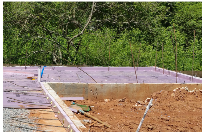
Under slab application. (Courtesy of Owens-Corning.)
