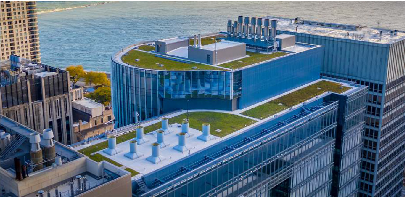
Figure 2 — Shown here is the 14-story base of a proposed 34-story building in Downtown Chicago. The architects developed a PMRA blue roof to meet the water retention and detention requirements of their building permit. The 14-story base of the building meets storm water management needs for the entire building through use of blue and green (vegetative) PMRAs. Photo Courtesy of American Hydrotech.
