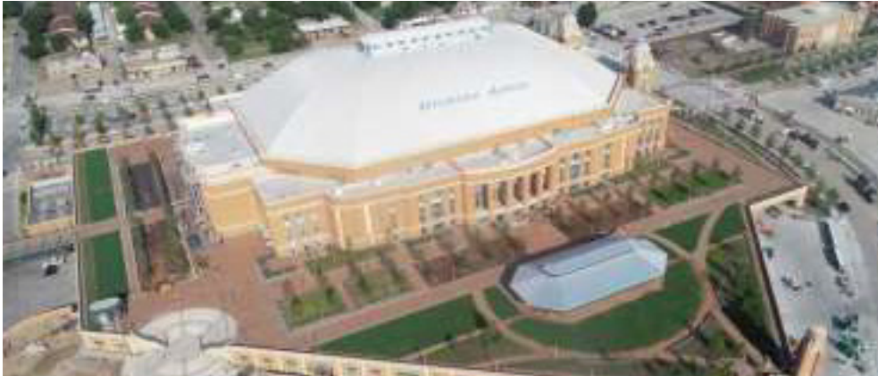
Figure 1 — The Dickies Arena in Fort Worth, Texas, is used for rodeo events. Partially encircling the arena, the Plaza Deck is a PMRA that is topped with walkways and a vegetative roof. Encompassing 9290 m 2 (100,000 sf), it serves as a practice area where handlers can warm up with their animals prior to rodeo events. Photo courtesy of Trail Drive Management Corp and Owens-Corning.
