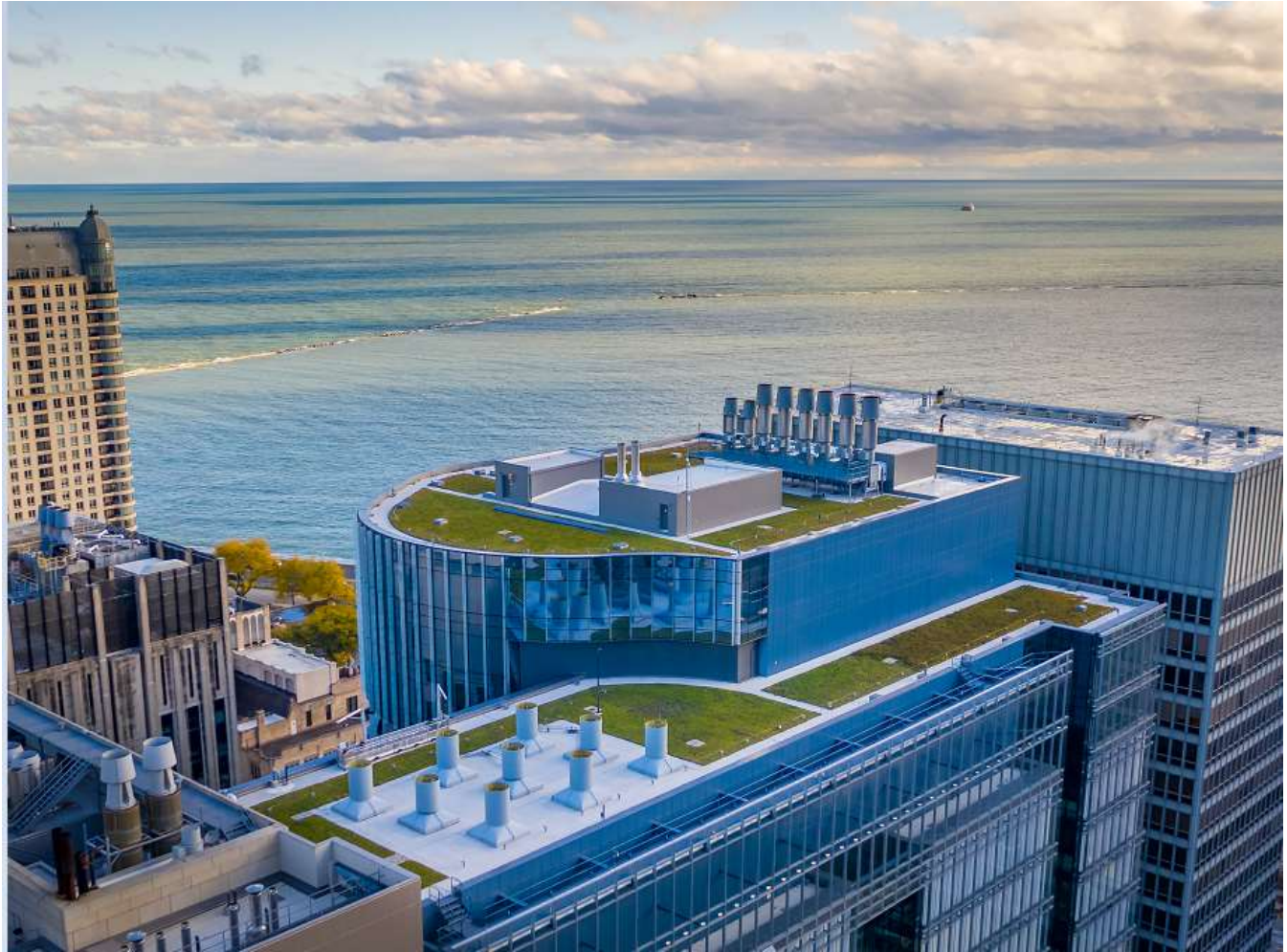
Figure 7. Shown here is the 14-story base of a proposed 34-story building in Downtown Chicago. The architects developed a PMRA blue roof, especially to meet the water retention and detention requirements of their building permit. The 14-story base of the building accommodates storm water management requirements for the entire building through the design of blue and green (vegetative) PMRAs. Photo Courtesy of American Hydrotech.
