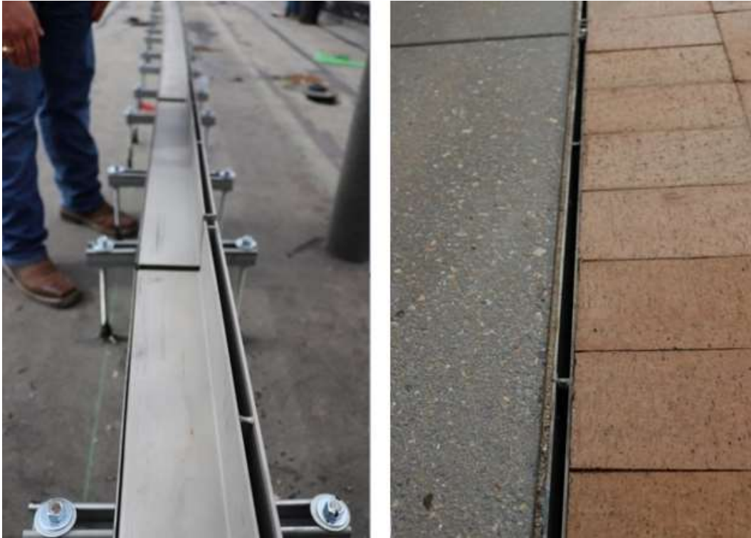
Figure 6. Slot drains channel the water to an engineered assembly of 261 drains (left). Tapered XPS insulation fills in the space between the roof membrane and slot drains. The completed linear drain shows how inconspicuous well-planned drainage can be (right). Photos Courtesy of Owens Corning.
