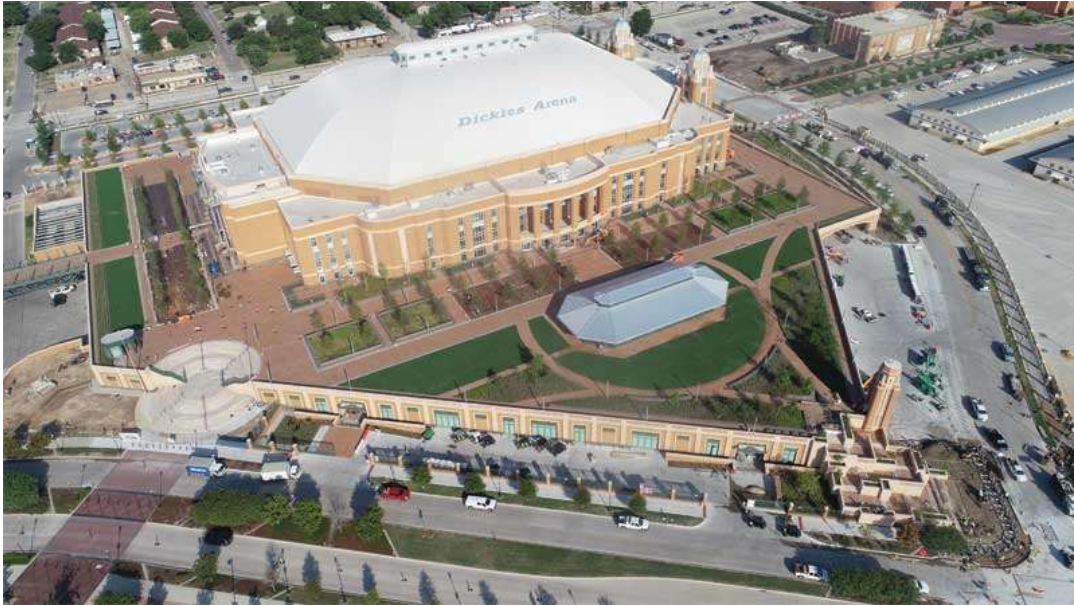
Figure 2. The Dickies Arena in Fort Worth, Texas, is used for rodeo events. Partially encircling the arena, the Plaza Deck is a PMRA that is topped with walkways and a vegetative roof. Encompassing an area of 9290-m 2 (100,000-sf), it serves as a practice area where handlers can warm up with their animals prior to rodeo events. Photo courtesy Trail Drive Management Corp and Owens-Corning.
