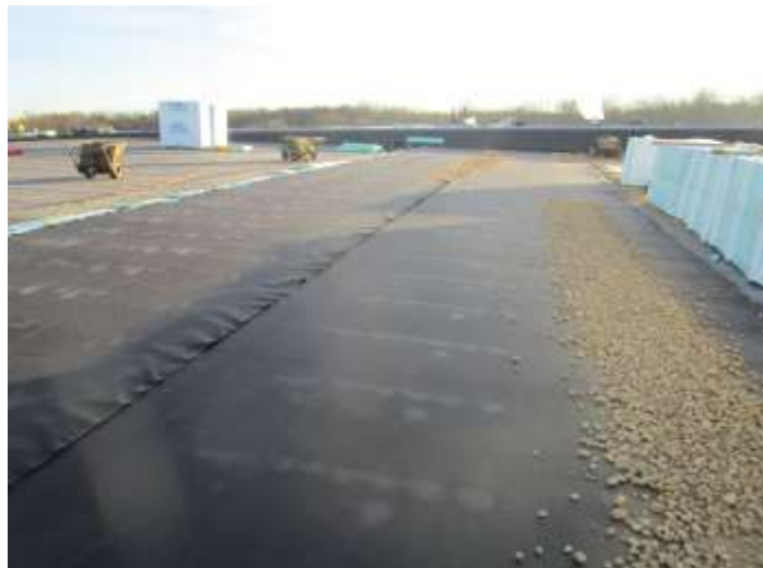
Figure 4. Type VI XPS with a compressive strength of 40 psi was adequate for the relatively light load on this PMRA. Photo Courtesy of Kingspan.
