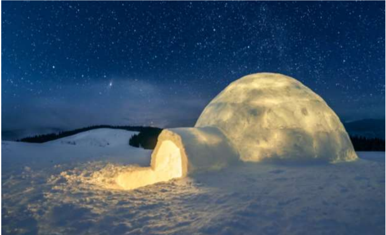
Figure SB1: The R-value of snow keeps the colder temperatures outside. Thirty inches of snow performs about as well as two inches of dry XPS. Most igloos don't survive a long freeze-thaw cycle, but snow blocks are readily available in some climate zones. (Adobe Stock)
