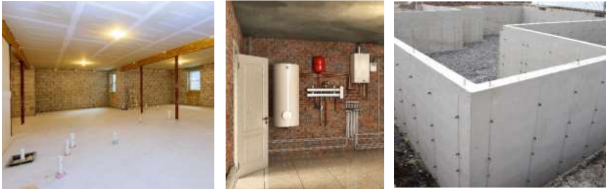
Figure 3: Basement walls can be made of concrete blocks ( left ), bricks ( center ) and other materials but most commonly are made of concrete ( right ). Basement walls need to be kept warm to protect them from the condensation of water vapor in the basement air space. (Adobe Stock)
