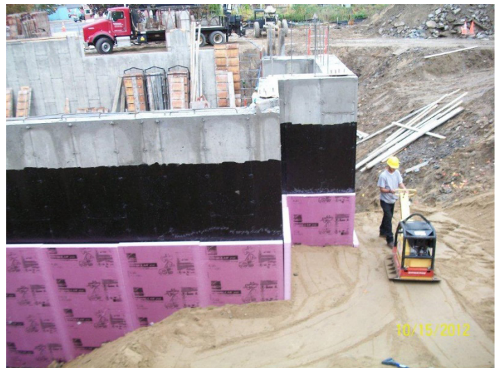
Figure 3: XPS Insulation is a key component of any basement wall assembly. The moisture resistance of XPS makes it ideally suited for below grade applications in the construction of habitable basements. (Courtesy of Owens-Corning)
