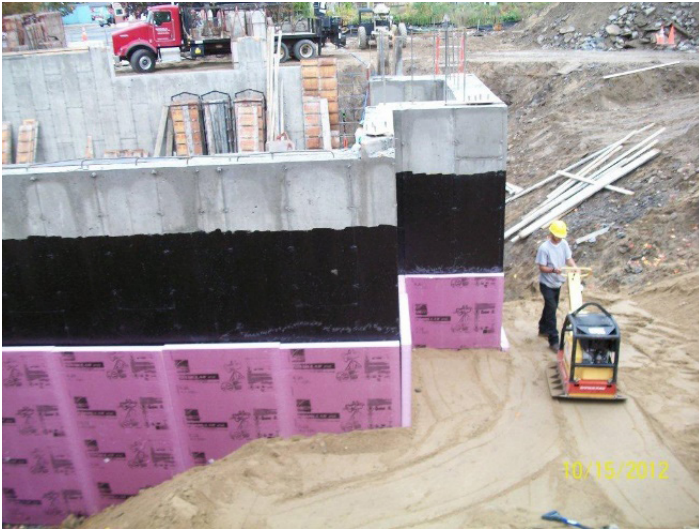
Figure 3: XPS Insulation is a key component of any basement wall assembly. The moisture resistance of XPS makes it ideally suited for below grade applications in the construction of habitable basements. (Courtesy of Owens-Corning)
