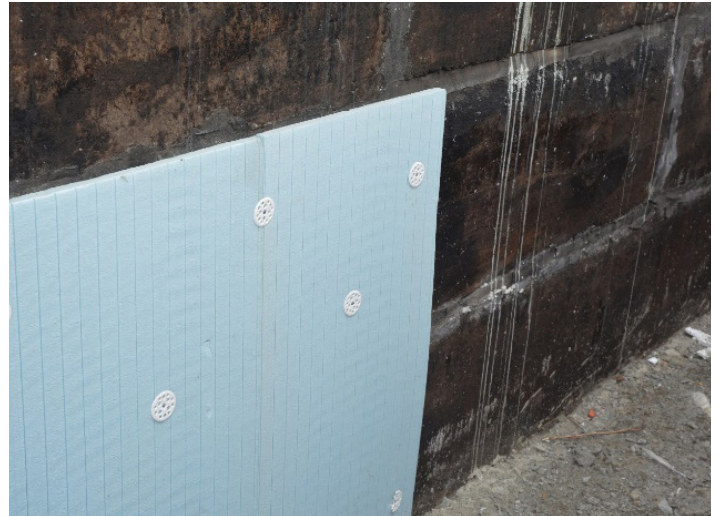
Figure 2: XPS insulation on exterior of basement wall showing damp-proofing, wall insulation and anchors outdoors. (Adobe Stock)
