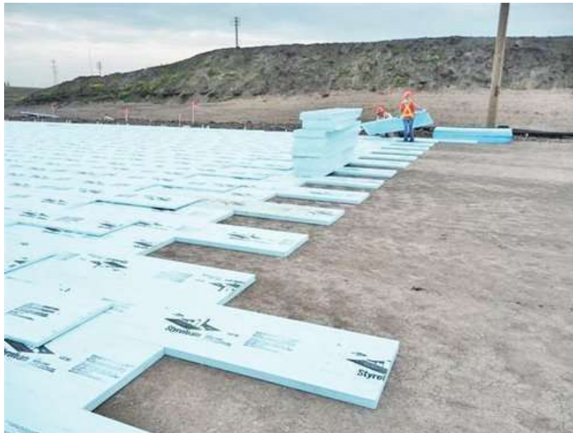
Figure 1 – RCPS is often installed beneath airfields in cold climates. (Photograph Courtesy of DuPont.)
