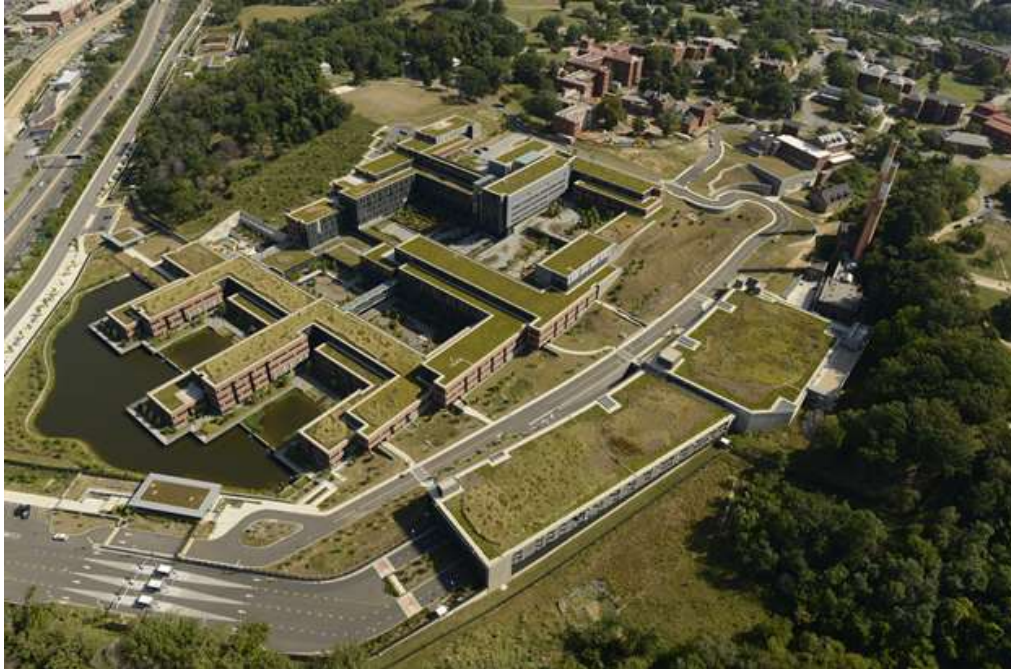
Figure 7 — Aerial view of U.S. Coast Guard Headquarters. XPS insulation must resist compressive loads from the weight of vegetative or “green” roofs. The appearance of U.S. Department of Defense (DoD) visual information does not imply or constitute DoD endorsement.
