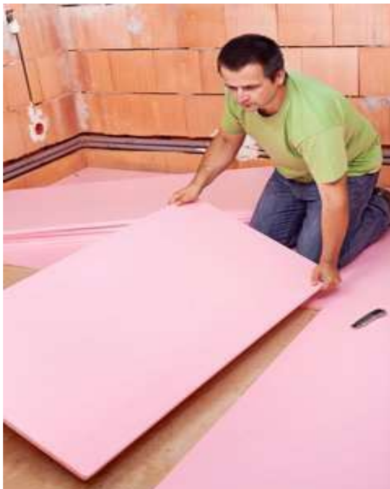
Figure 3 — RCPS can be used in horizontal floor applications as well as vertical wall applications.
