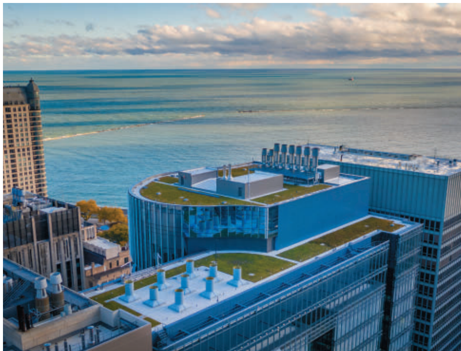
Figure 1. The architects of this building in downtown Chicago developed a protected membrane roof assembly (PMRA) blue roof, especially to meet the water detention requirements of their building permit. The 14-story base of the building accommodates storm water management requirements for the entire building through the design of blue and green (vegetative) PMRAs.
