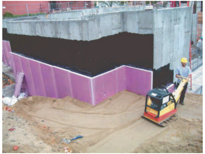
Figure 3. Rigid, cellular polystyrene foam boards can be used in horizontal floor applications as well as vertical wall applications.
