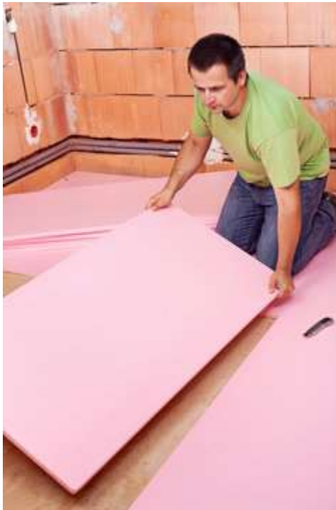
Figure 3. RCPS foam boards can be used in underslab as well as vertical wall applications.
