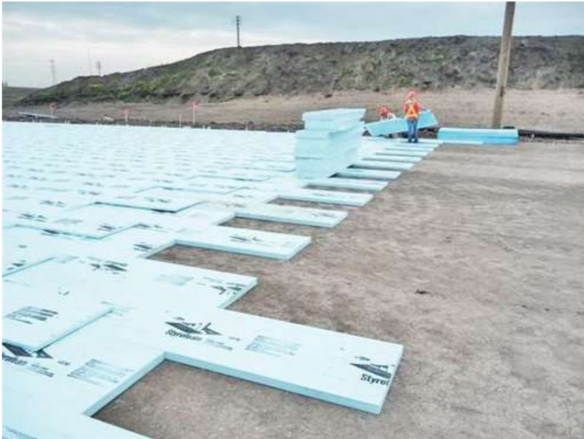
Figure 1. RCPS foam boards are often installed beneath airfields in cold climates. Photograph courtesy of DuPont.
