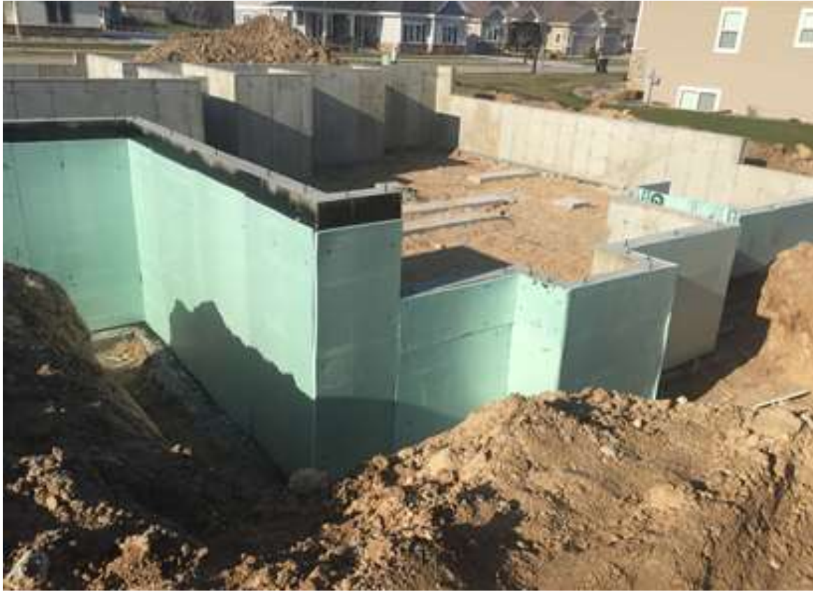
Figure 2. RCPS foam boards are often installed in below-grade applications for habitable basements. Photograph courtesy of Kingspan.
