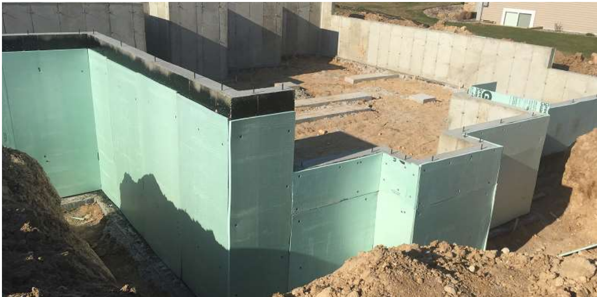
Figure 2: Exterior insulation and damp-proofing or waterproofing along with effective drainage helps prevent water intrusion into the basement. (Courtesy of Kingspan.)
