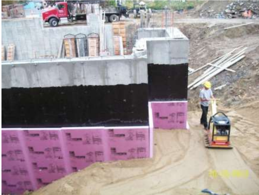
Figure 11: XPS Insulation is a key component of any basement wall assembly. The moisture resistance of XPS makes it ideally suited for below grade applications in the construction of habitable basements. (Courtesy of Owens-Corning)
