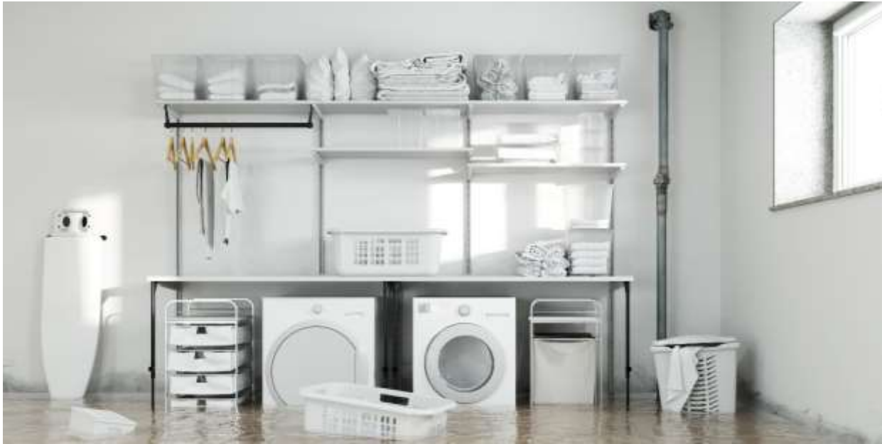
Figure 4: This basement has a water management problem. A habitable basement must have effective environmental separation, meaning bulk water must not penetrate the interior of the basement. (Adobe Stock)
