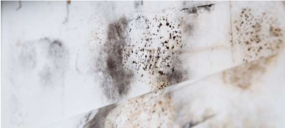
Figure 6: If basement walls are not insulated from the outside, the wall temperature could drop below the dew point. Moisture condensation in the dark spaces behind interior insulation and sheet rock creates conditions that favor the growth of mold and mildew. (Abohe Stock)
