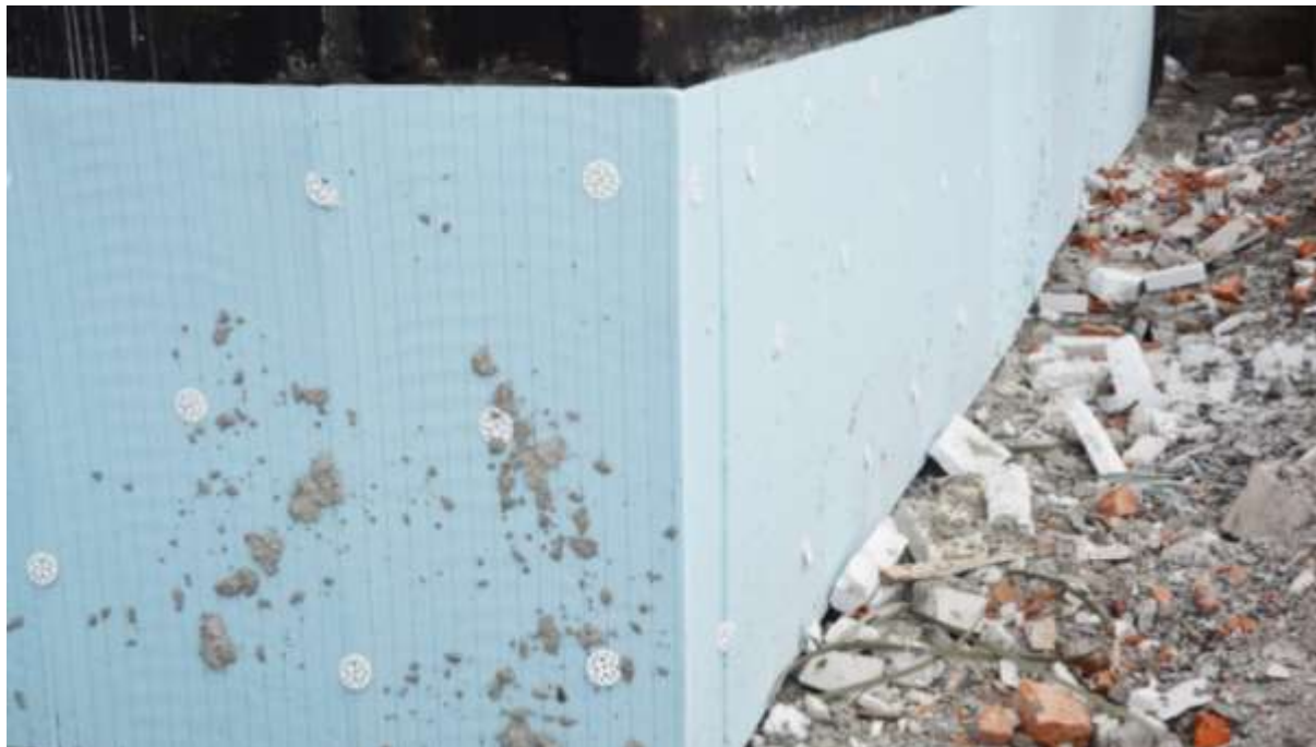
Figure 10: XPS has the toughness and moisture resistance suitable for direct contact with surrounding debris. Here the XPS insulation protects the waterproofing membrane. (Adobe Stock)
